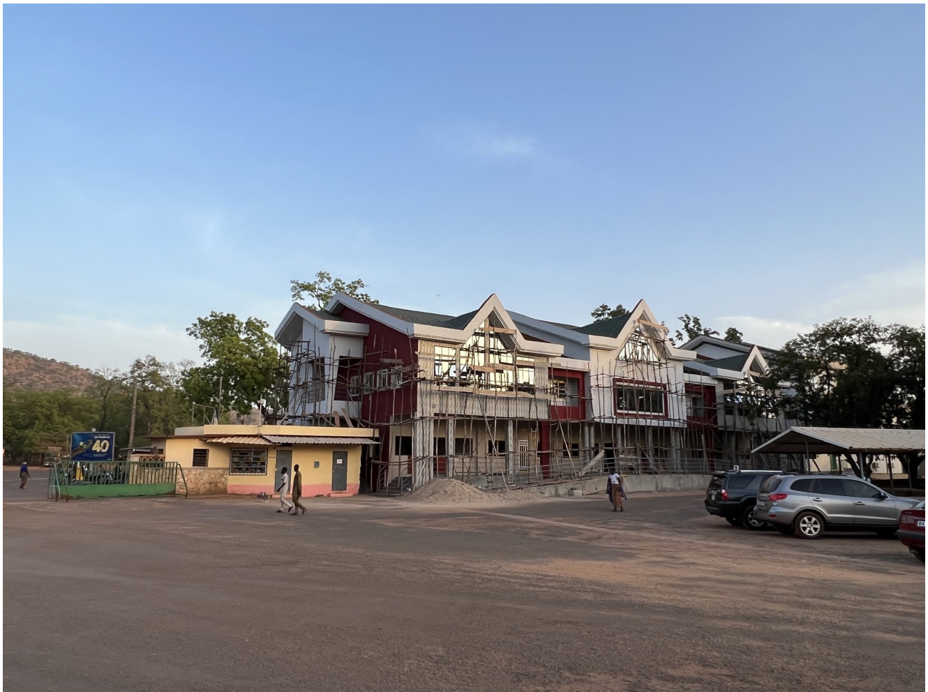
Renovation of clinic building
